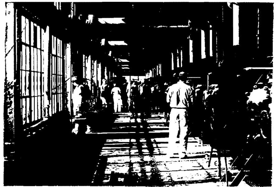
TURNER VALLEY PLANT COMPRESSOR BUILDING
