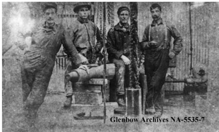
Drilling crew in the drill shack on Dingman #2 well , just to the west of the Dingman #1 Discovery Well, Turner Valley, 1914. Joe Brown, far right, is getting ready to sharpen a fish tail bit before lowering it down the well. Heavy chains, strung from the drilling rig framework, were necessary to allow the heavy equipment to be moved about the rig floor. With the permission of the Glenbow Archives. Image Number NA-5535-7 (Copied from PA-3296).
