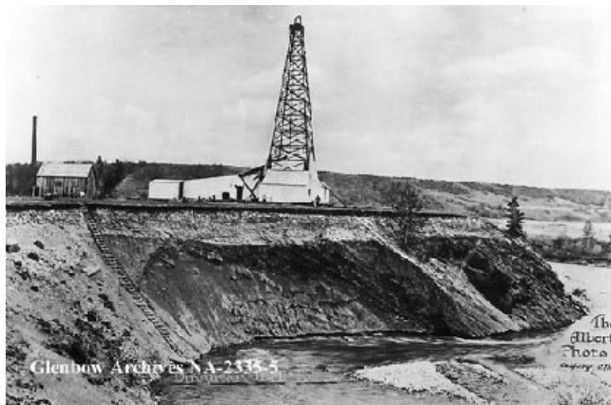
Dingman #2 wellsite with cable tool rig, just above the Sheep River and south of Turner Valley, Alberta, 1914. The well was later renamed Calgary Petroleum Products #2. Photo by the Alberta Photo Company. Several features are notable. First is the distinct layering present beneath the rig. From top to bottom these are: soil layer (black, approx. one foot thick); unconsolidated gravel layer (light coloured with obvious pebbles and cobbles – of glacio-fluvial origin); and finally steeply dipping deformed shales and thin sandstones of the Late Cretaceous Alberta Group that core the surface anticline at Turner Valley. The river seems to be a lot closer to the cliff than it is now – such movements of the channel are a problem with the gas plant site overall. The current burning seep that can be visited near the plant is in these riverside shales but is apparently sourced from a cracked casing in the wellbore of the #2 well, rather than being a genuine subsurface seep. With the permission of the Glenbow Archives. Image Number NA-2335-5.
