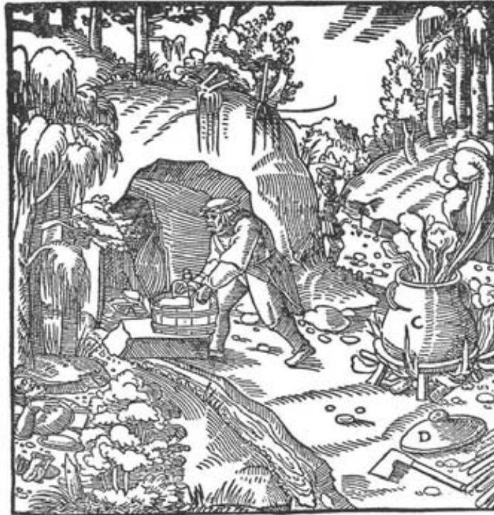
Fig. 15. Crude-oil winning and refining (after Agricola, De re metallica , 1556).
