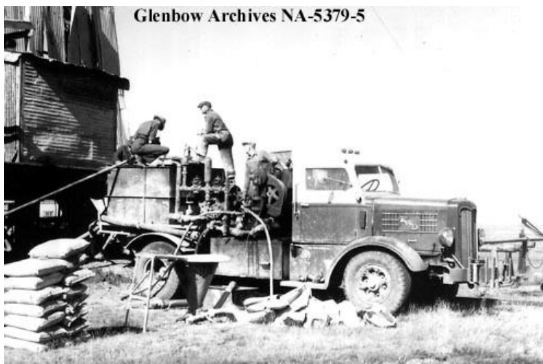
Standard Oil of British Columbia Eyremore, Alberta 1942. Halliburton truck running cement (photo NA-5379-5 courtesy Glenbow Archives)
