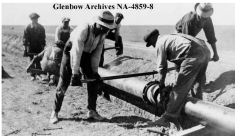
Photo 2 - Construction of gas pipeline from Turner Valley (Source: Glenbow Archives)
