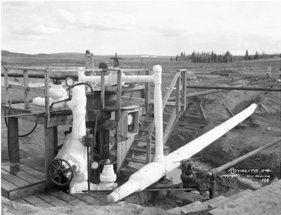
Photo18: Later photo that includes the pressure monitoring charts and full frosted wellhead. Source: Glenbow Archives.
