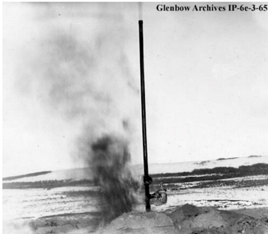
Photo 2: Royalite No. 4 flames from cellar and out the 6-inch valve can be seen at floor level with a flow tee below. The 25-foot joint above is the "handling joint". Source: Glenbow Archives.
