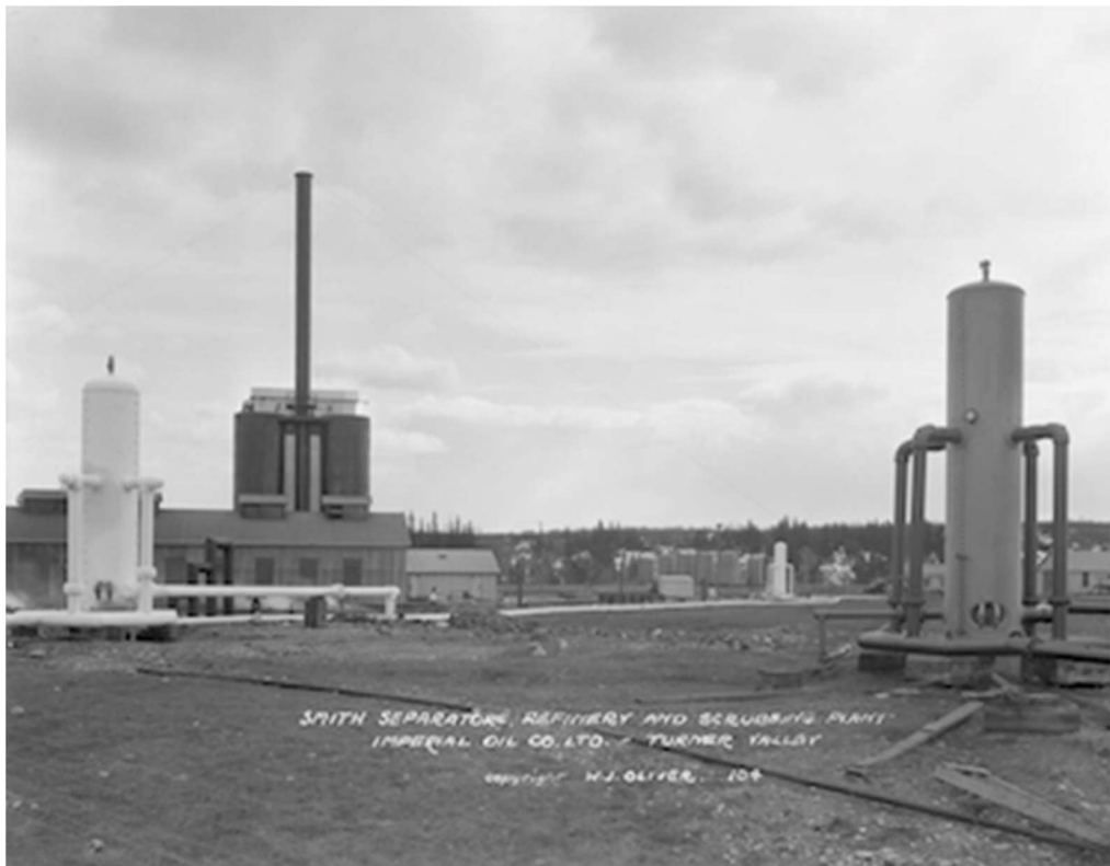
Photo 21: Royalite's first scrubbing plant with 3 Smith separators in view. Source: Glenbow Archives.
